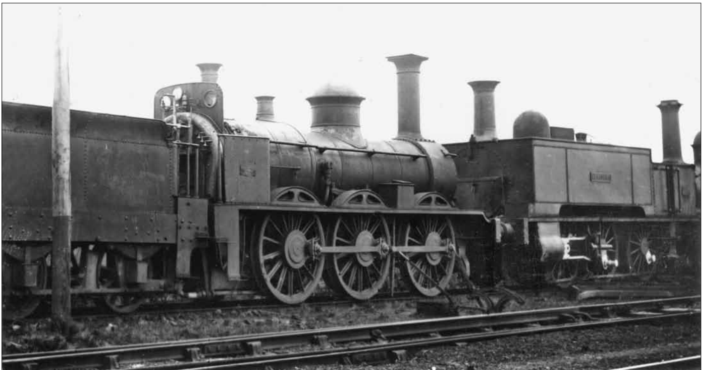
Another Boulton's Sidings product to appear on the N&BJR was an 1847 Longridge-built tender 0-6-0 named Cotton, late of the L&NWR, which was provided to contractors John Aird & Son at Blisworth around 1870. At this time, construction of the N&BJR had just restarted from a point in a field west of Towcester and was advancing towards a junction with the L&NWR at Cockley Brake. As with the 'Sharpie' six years earlier, Cotton's main function would have been with the contractor but there is every possibility that the locomotive may have been pressed into service to assist on the newly opened section. Boulton had a few of these locomotives, one of which is pictured here in the yard at Ashton, in the company of another of his diverse collection of rebuilt antiques.
