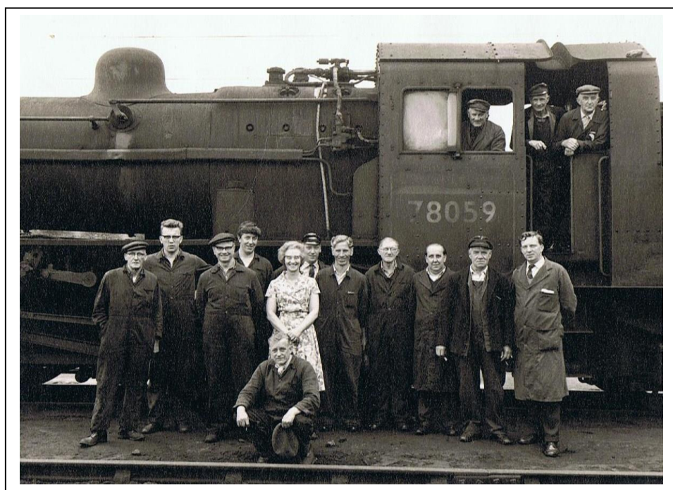
Nr. 78059 was the last steam loco to be allocated to Nuneaton shed. It is seen here at the time the shed closed on 6 th June 1966. It stayed on a further three weeks to clear stores, empty the coal and ash plant, before being sent away to Crewe South shed. The shed staff are: on the ground in front of the engine – George Brookes, Edwin Holmes, Harry Gunn, Alan Burnham, (fitters) (Kneeling) – George Hall, fitter’s mate; Hilda Randle, office clerk, ----fireman, Ernie Morris, office clerk, Jack Green, fitter; ---- running shed foreman’s office clerk, Don Foulds, Driver; Bill Lowe, running shed foreman; On the footplate: Albert Harris, Alf Drake, drivers and Charlie Woodford, fitter. (Charlie Woodford Collection)
