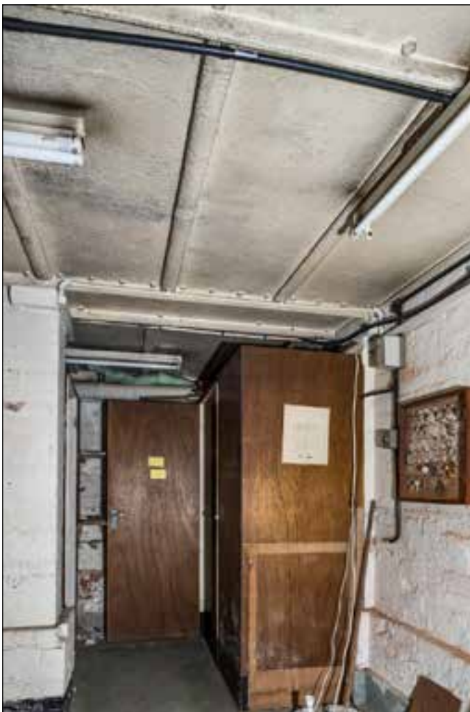
Figure 30: The iron ceiling found in the basement towards the centre of the building on the western side. ©Historic England DP164946.
