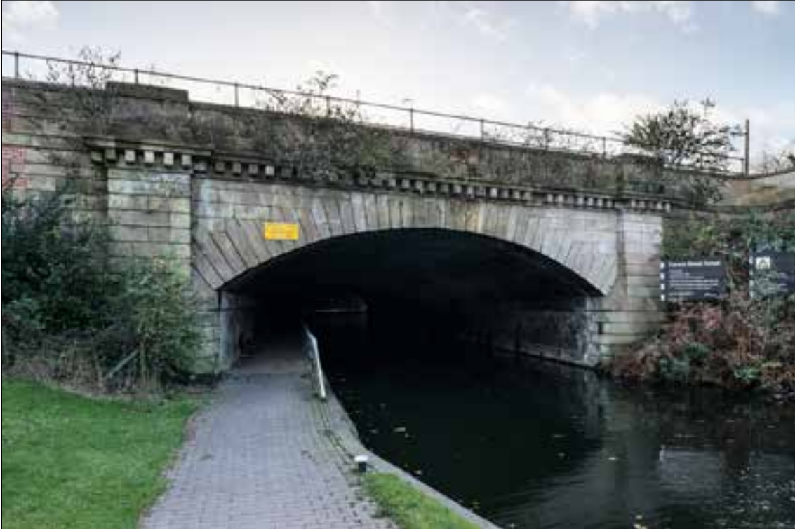
Figure 38: The bridge carrying the lines into Curzon Street over the Digbeth Branch Canal, looking south. ©Historic England DP164960.
