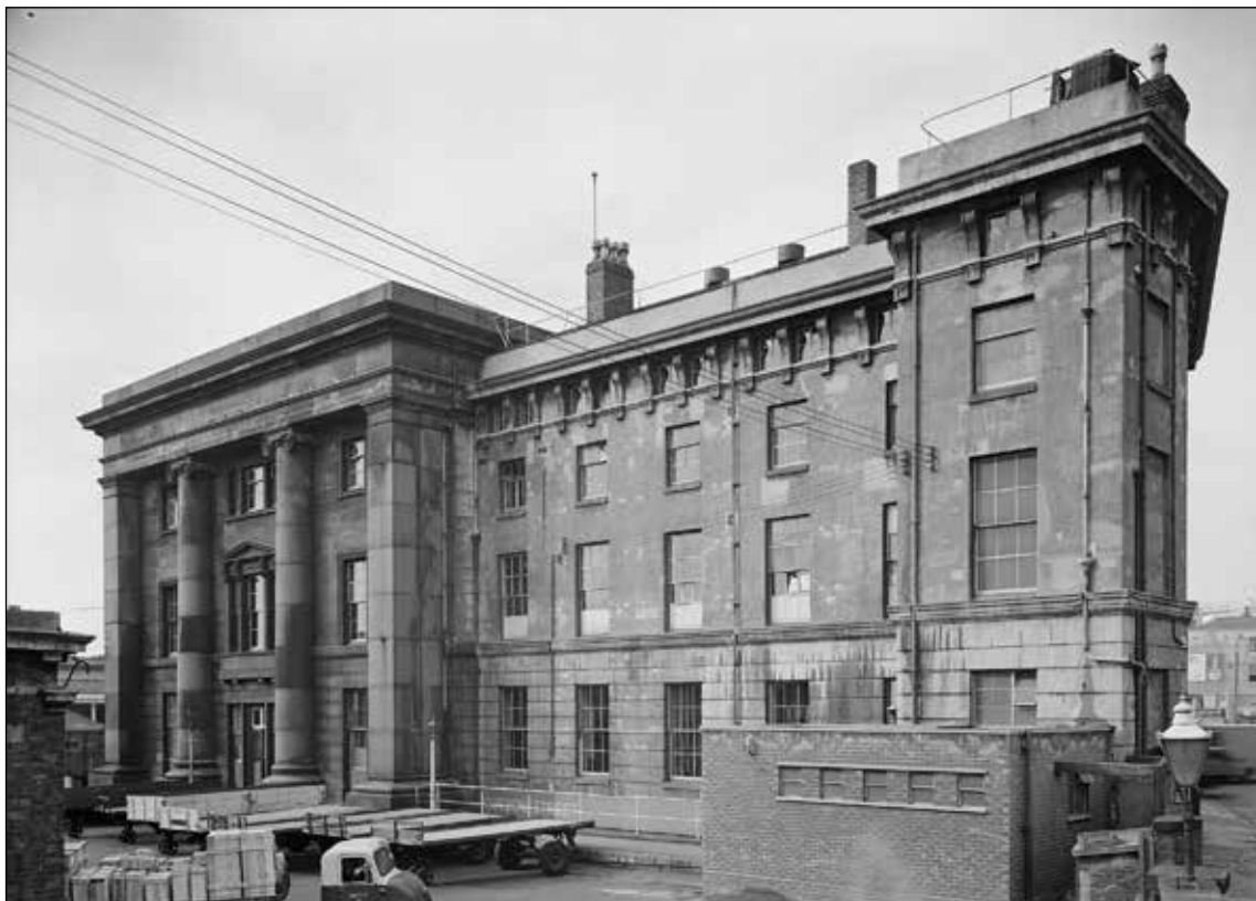
Figure 6: The rear of the Principal Building, clearly showing the 1841 hotel addition with the wing for bathrooms and WCs on the right. 1966. ©Historic England Archive bb64_02100.
