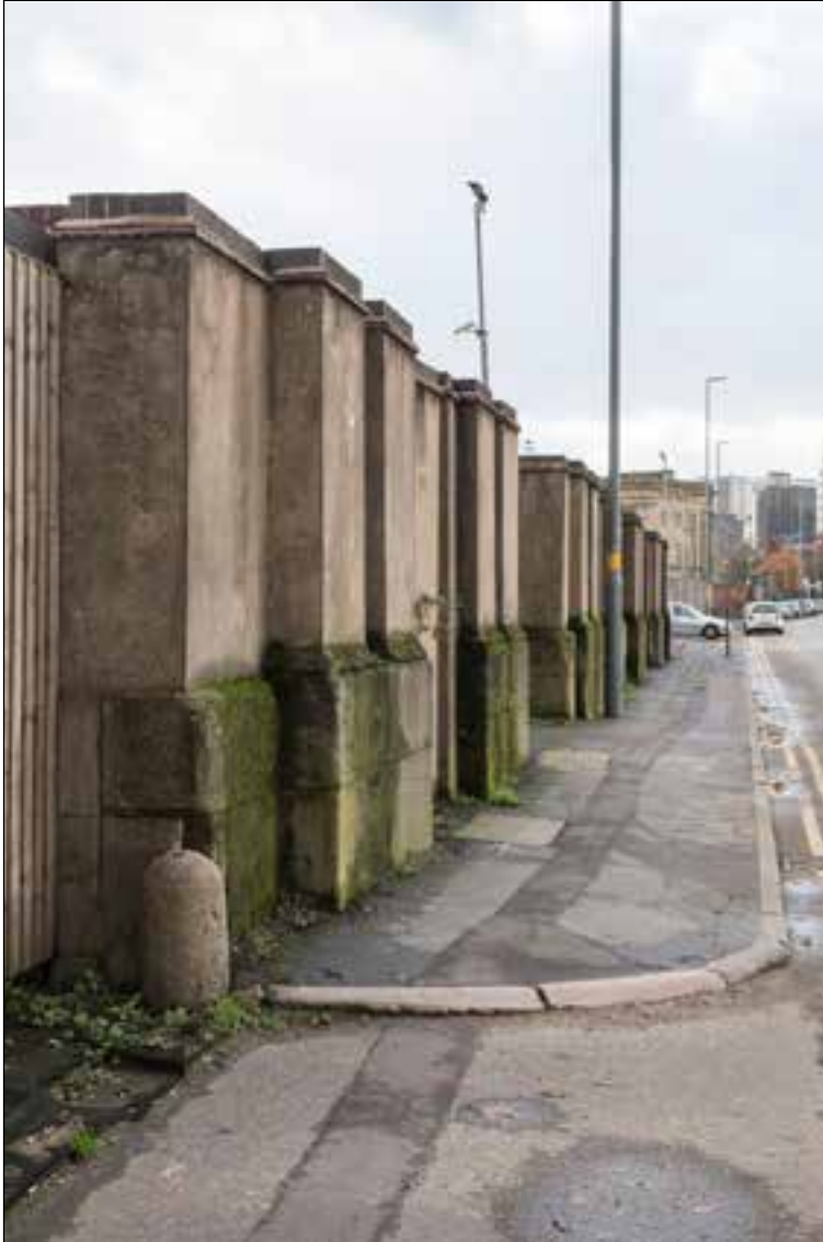
Figure 36: The remains of the screen wall, looking towards the 1838 Principal Building. A granite gate pier protector and curved curb stones to the entry remain. ©Historic England DP164955.
