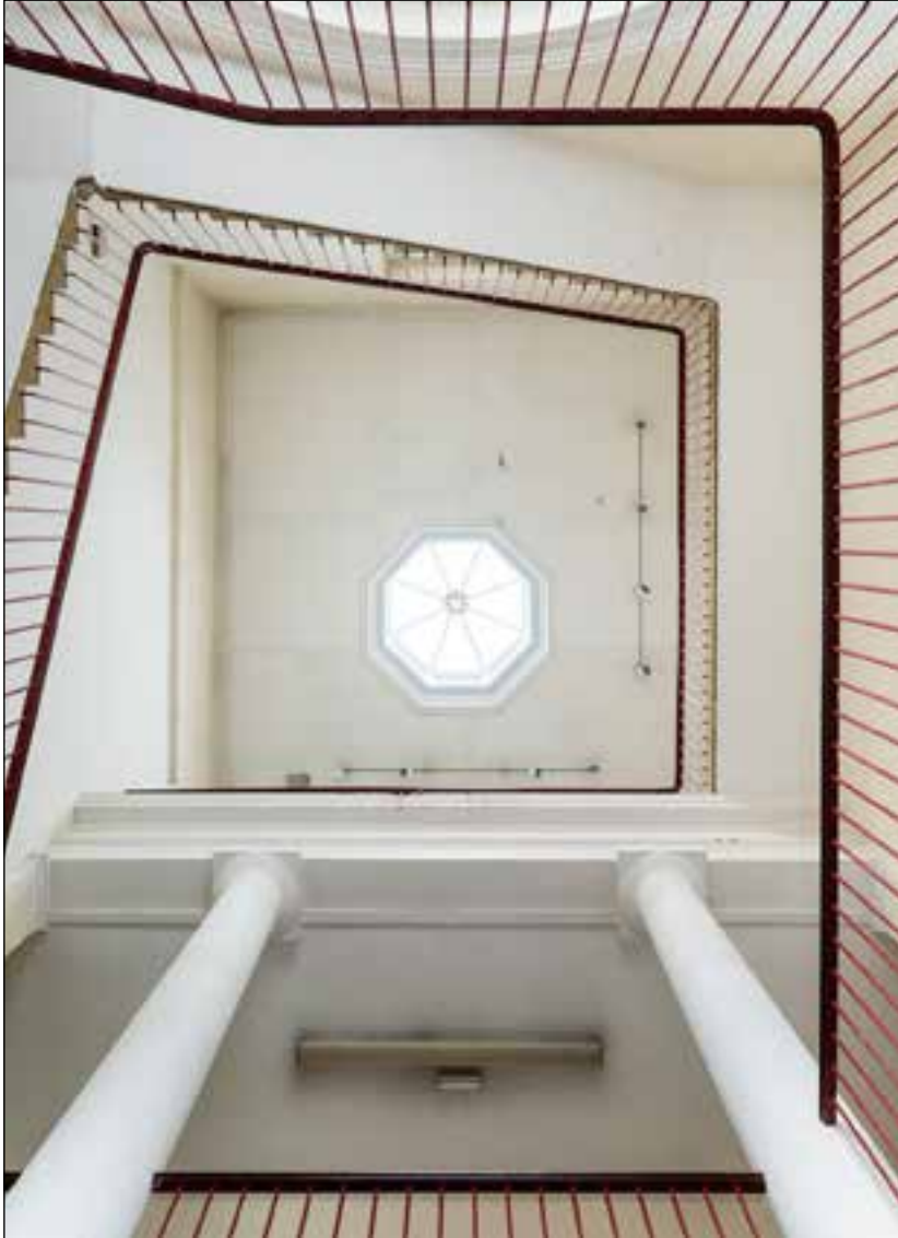
Figure 21: Looking up towards the skylight in the entrance hall. ©Historic England DP164919.
