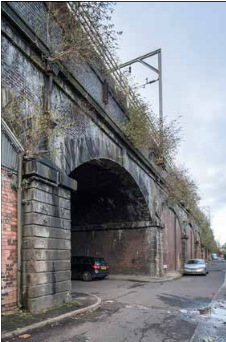
Figure 41: The GJR viaduct seen from Viaduct Road, looking east. ©Historic England DP164965.
