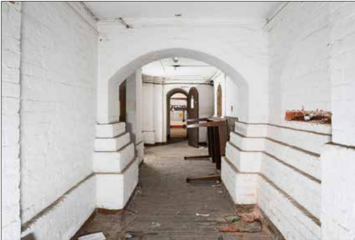
Figure 29: The basement, showing the tiered construction of the walls. ©Historic England DP164947.
