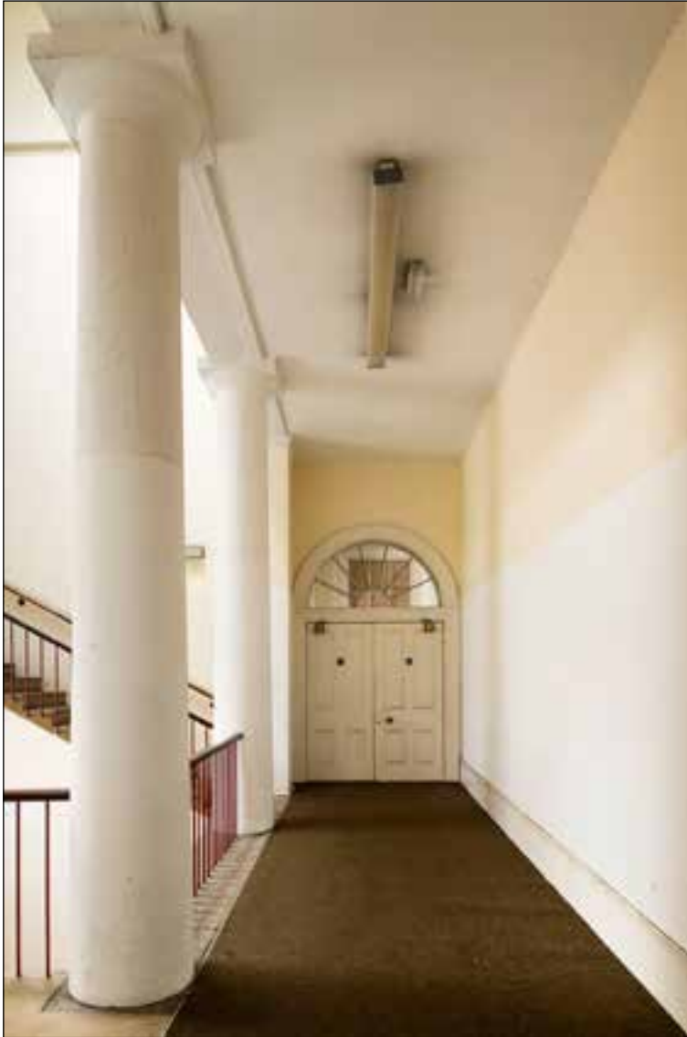
Figure 23: The first floor landing showing the doors leading to the central corridor. ©Historic England DP164928.
