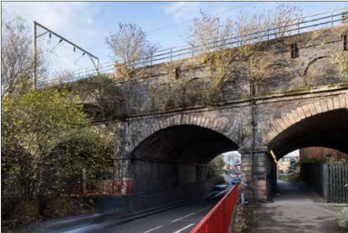
Figure 40: The Grand Junction Railway viaduct looking north where it crosses Lawley Middleway. The additional arches added above the cornice in 1893 to raise the GJR route sufficiently to avoid it crossing the goods lines on the level are clearly evident. ©Historic England DP164962.
