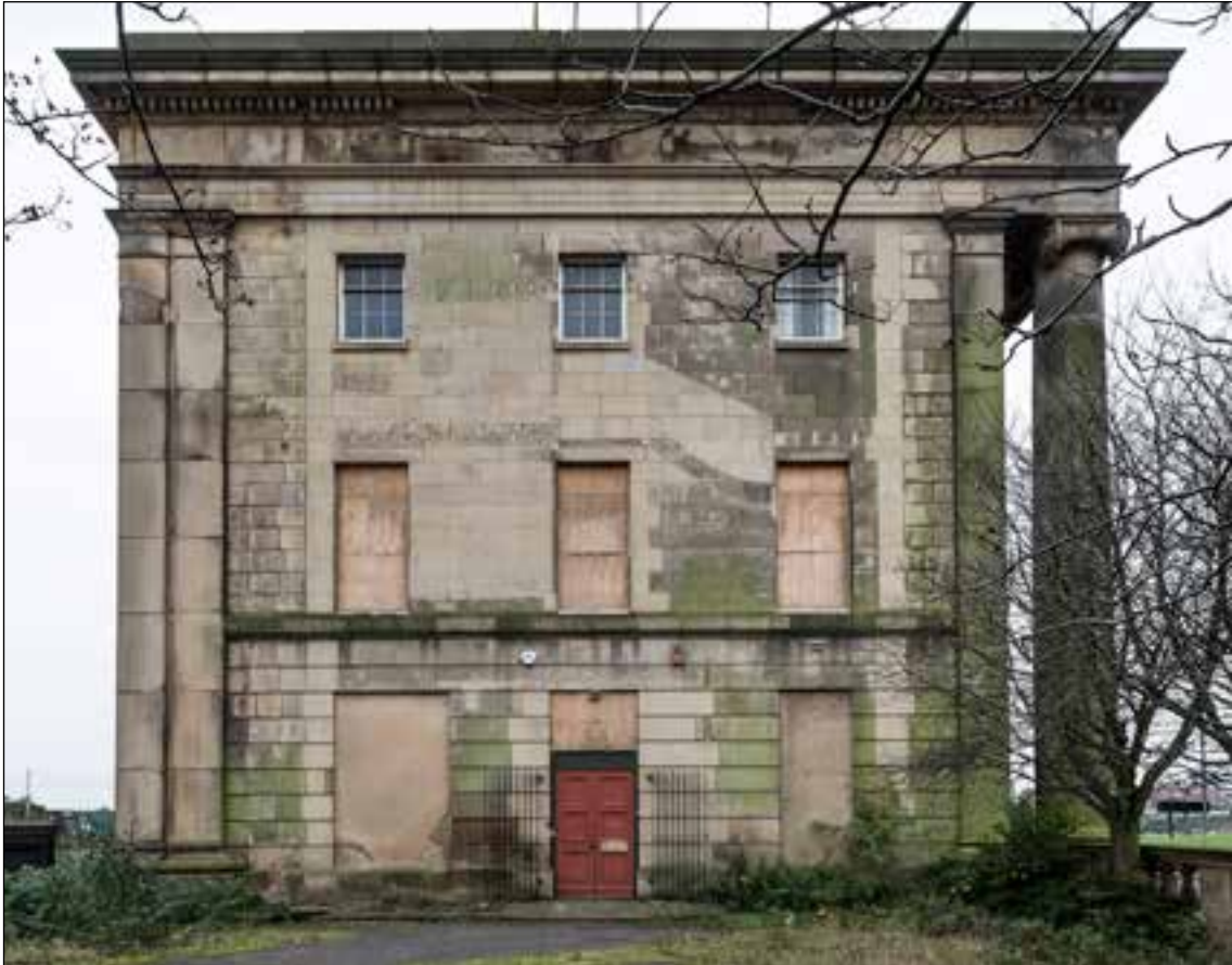
Figure 18: The north façade of the Principal Building. ©Historic England DP164913.
