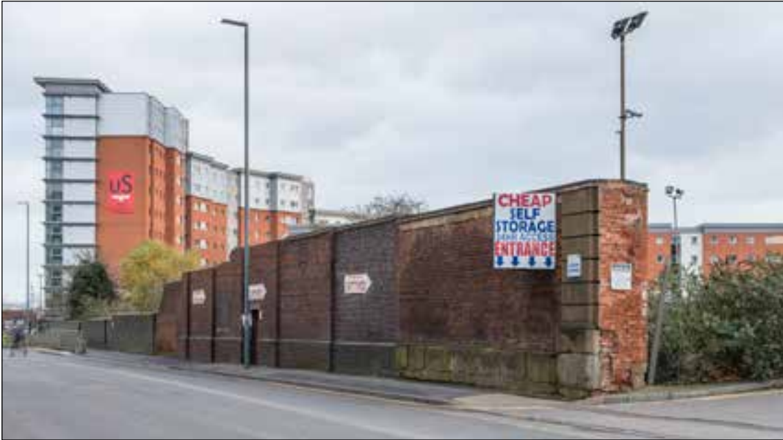
Figure 37: The most easterly stretch of the boundary wall of the Curzon Street site. The section of wall on an ashlar base may well be contemporary with the GJR screen while that beyond employs bands of the blue engineering bricks much favoured by the LNWR and incorporates a blocked window from the accumulator tower. ©Historic England DP164958.
