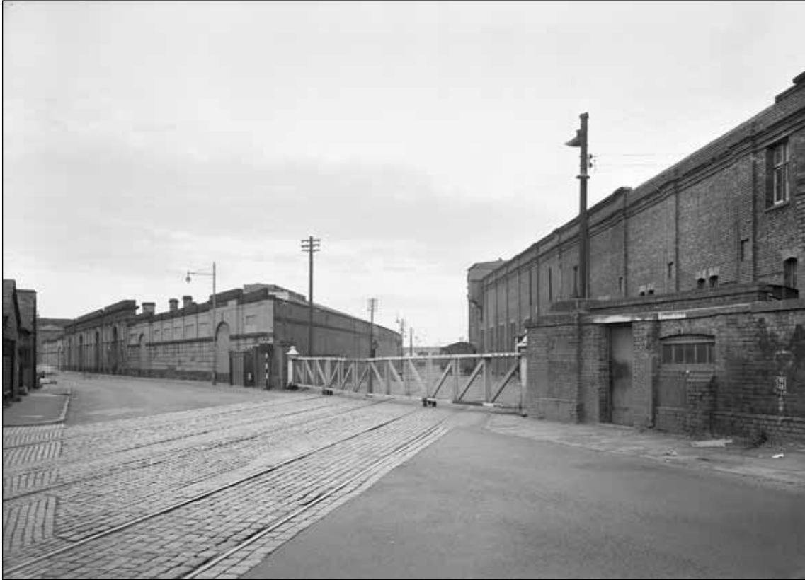
Figure 11: The level crossing over Curzon Street with the tracks leading to the original L&BR goods depot, located behind the photographer, and showing the position of the GJR screen wall. 1966. ©Historic England Archive bb64_02093.
