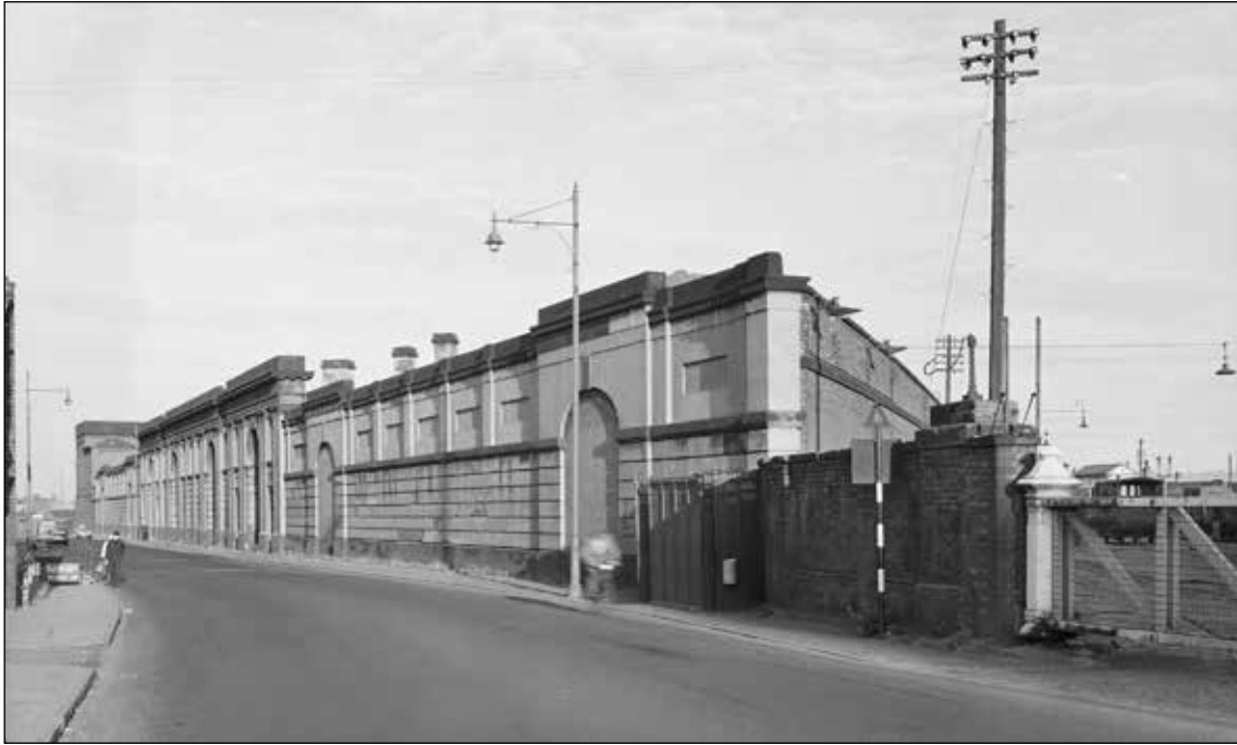
Figure 9: The full extent of the screen wall of the Grand Junction Railway station looking east along Curzon Street with the accumulator tower visible on the far left. 1966. ©Historic England Archive bb64_02091.
