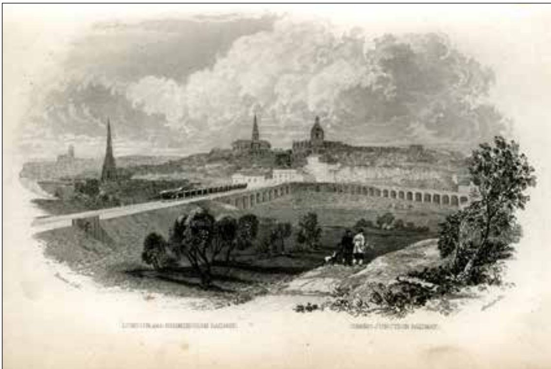
Figure 39: The converging London & Birmingham Railway and Grand Junction Railway viaducts with Curzon Street station visible in the background. From Drake's Road Book of the London & Birmingham and Grand Junction Railways, 1840.
