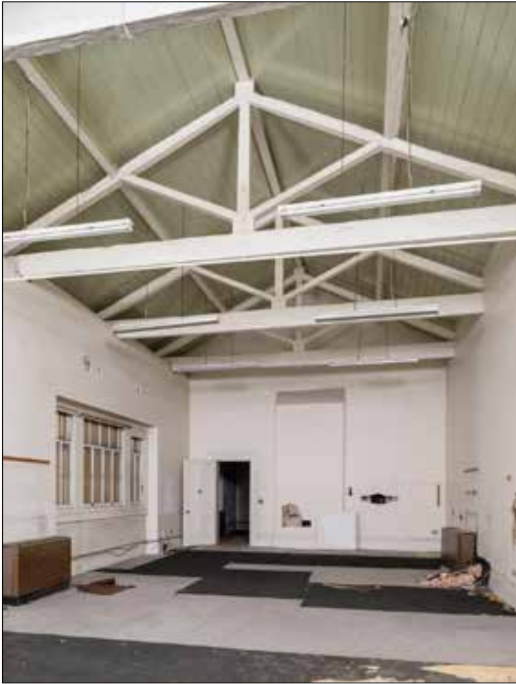
Figure 27: Room 2 on the second floor, with its exposed king post roof trusses. A large room with no function shown in the 1837 drawings, possibly occupied by clerks. ©Historic England DP164939.
