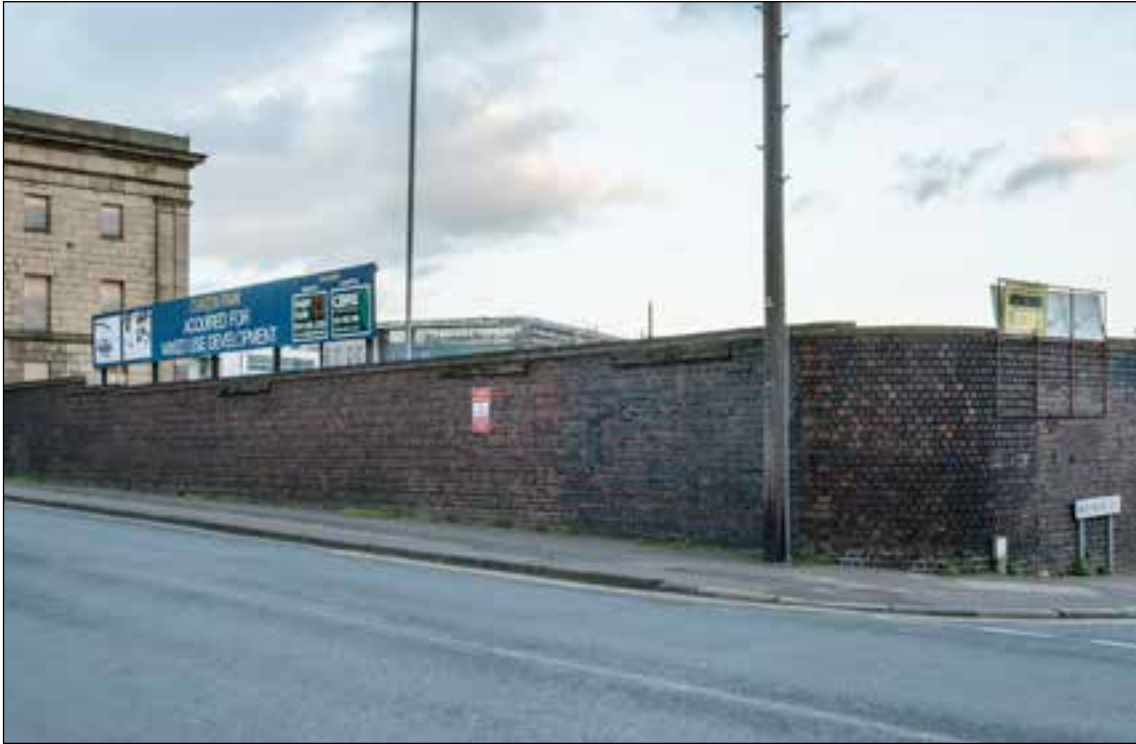
Figure 33. The boundary wall of the goods station, south of the 1838 building, with the sills of windows formerly part of buildings constructed abutting the wall. ©Historic England DP164951.
