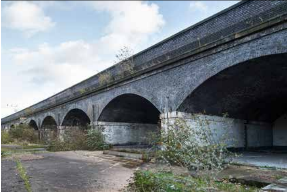
Figure 42: The north side of the GJR viaduct, as widened in blue engineering brick in 1893. ©Historic England DP164969.
